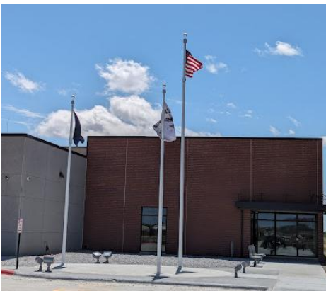
Public entrance, northwest corner of building
