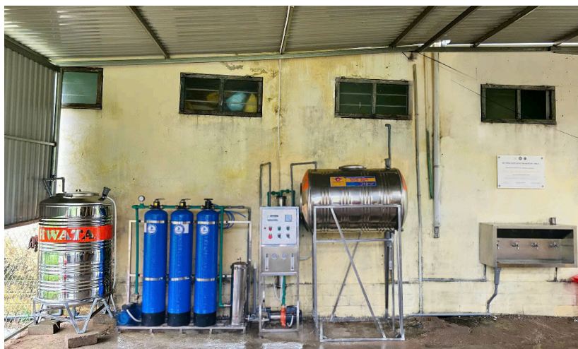
The two RO systems recently installed in Ta Long Kindergarten and Dakrong Primary School No. 2 by COV.
