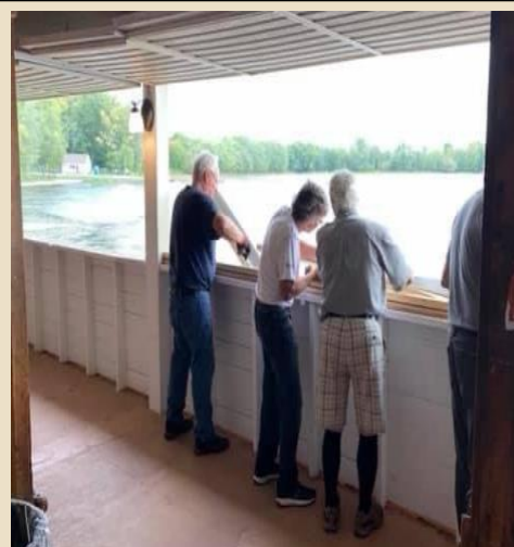
Kiwanians feeding the geese...oops I mean installing new windows.
