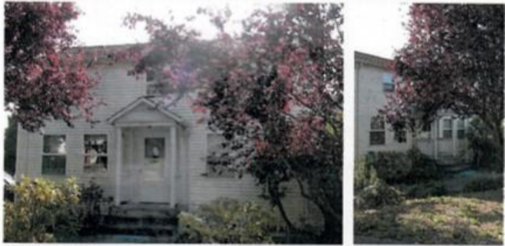
Front of Kiwanis House, west side facing 66th West
