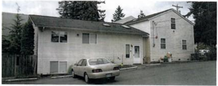
North side of Kiwanis House and parking lot
