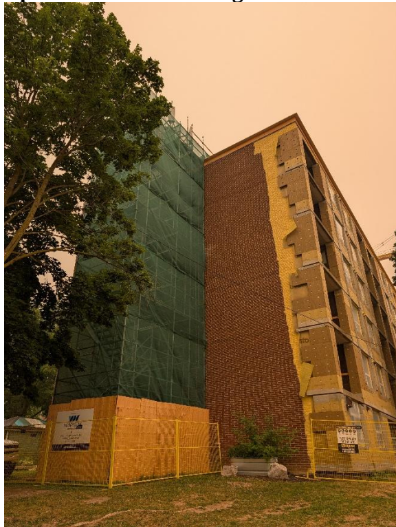
Exterior scaffolding and repairs at 59 Cedar Street North
