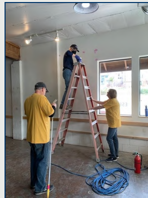
Yes, a Kiwanian up on the ladder patching holes
