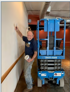
Pat Donaghey patching holes
